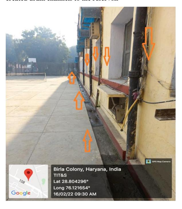
The heavy flow of rainwater from roof travels through these meandering drains (to avoid squalor) to the reservoir
