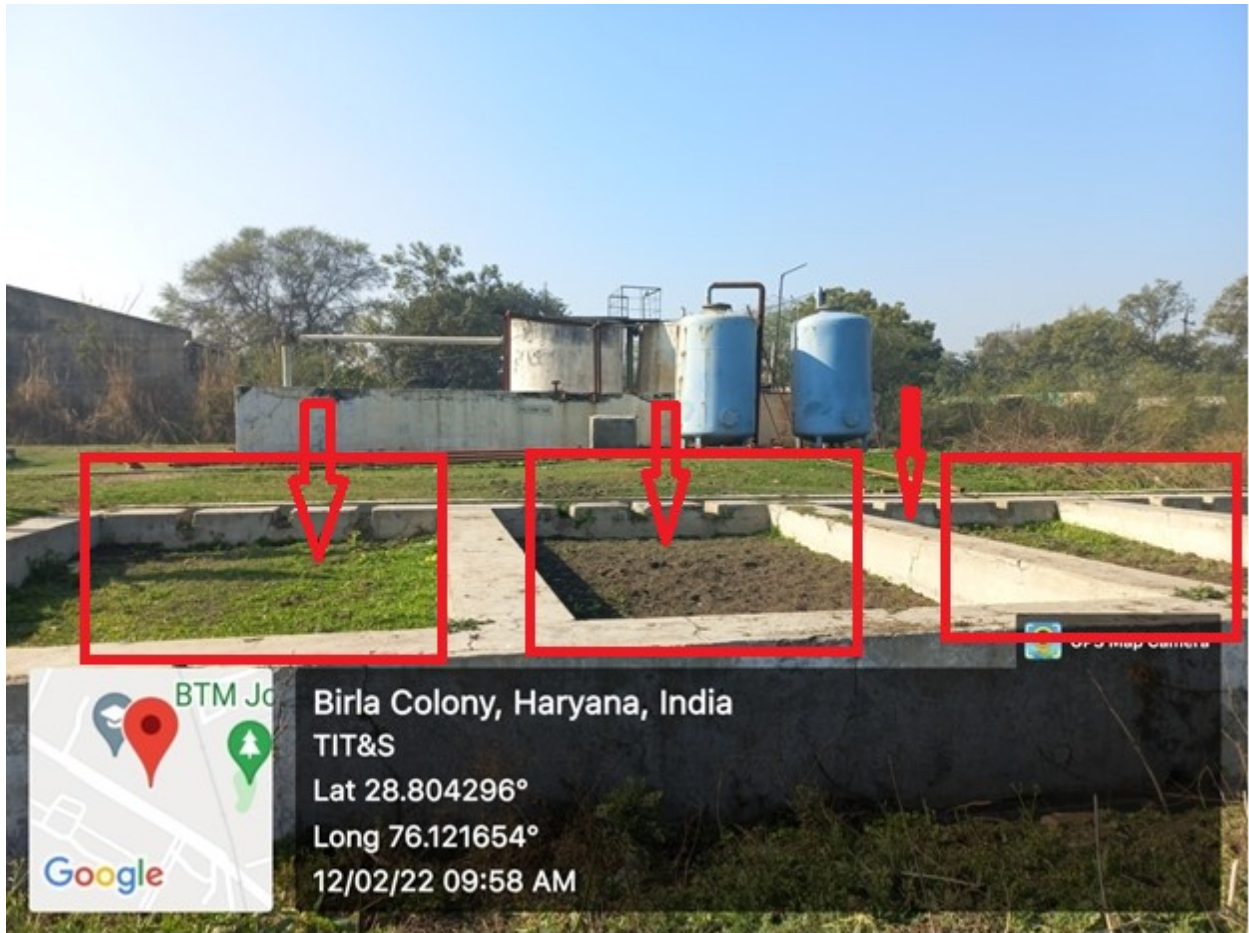
Open ground recharge near the STP
