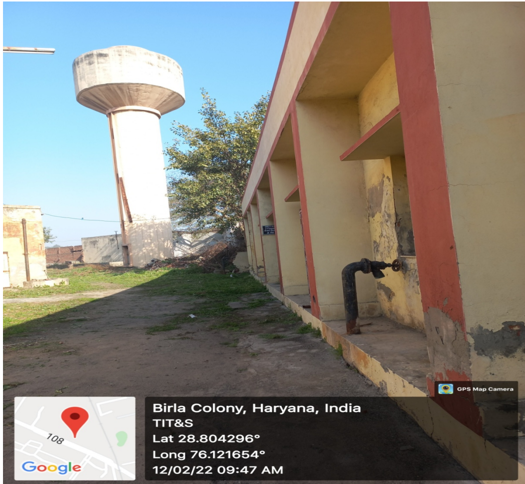
Water tank and distribution system
